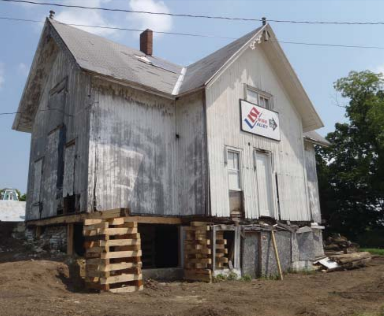
BullsEye Construction took down part of the 1930's foundation and installed new beams at the sw corner
