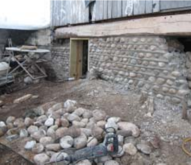
The west outside of the foundation is being restored to match the east side, using cobblestones from the Bonine House front yard
